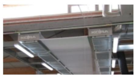
The ARB can be easily mounted in any workshop with a very ittle effort. Only a free area is needed. Further construction or flooring measres are not necessary. Using our special support frame set, the ARB is mounted anywhere regardless to the conditions of the site
