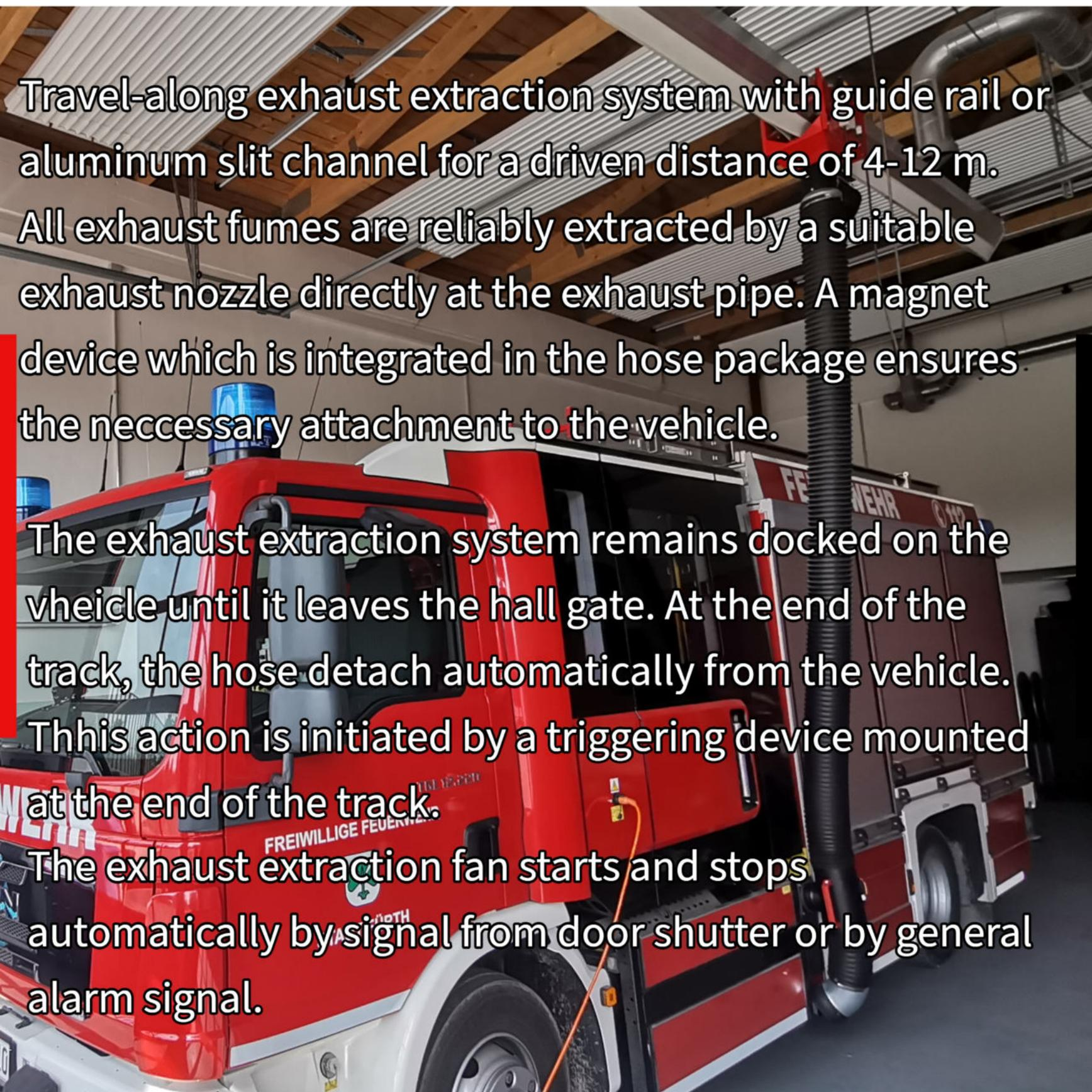
Travel-along exhaust extraction system with guide rail or aluminum slit channel for a driven distance of 4-12 m. All exhaust fumes are reliably extracted by a suitable exhaust nozzle directly at the exhaust pipe. A magnet device which is integrated in the hose package ensures the necessary attachment to the vehicle.
